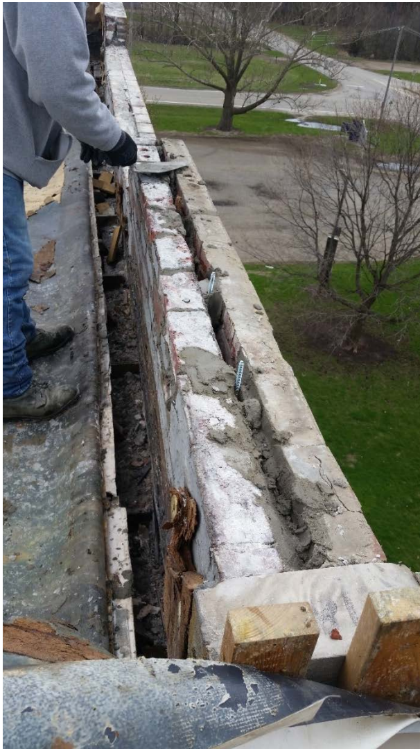
View of south parapet wall from 2016 showing the parapet construction
